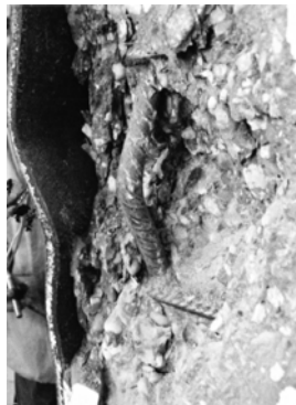
Figure 2.1: Buckling of longitudinal reinforcement by failure of column [2]
